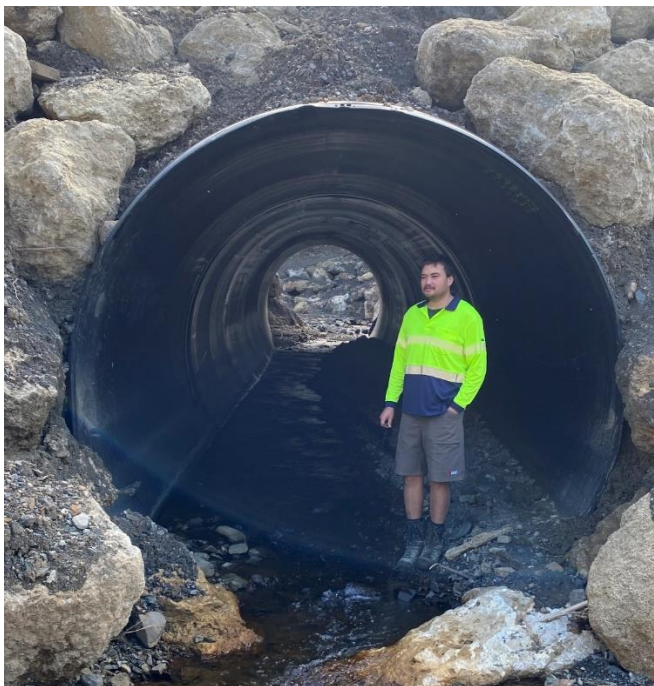
Figure 1: The new Allen Road culvert in Gwavas Forest. This was designed for greater than a 1:50 year flood event which not only increased flood resilience but allows for sufficient embeddedness which ensures passage for fish.
