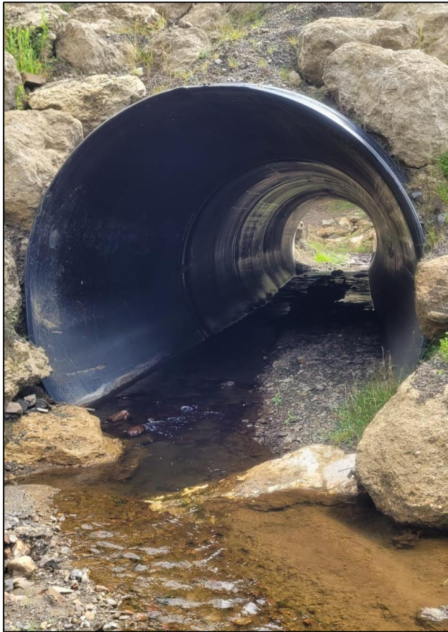
Figure 21: Allen Road culvert, Gwavas Forest. This culvert was replaced after Cyclone Gabrielle, and over- spec'd to a 1-50 year size. This has allowed for the bottom to be embedded, which retains bed material within the culvert and enables passage for both climbing and swimming fish species.
