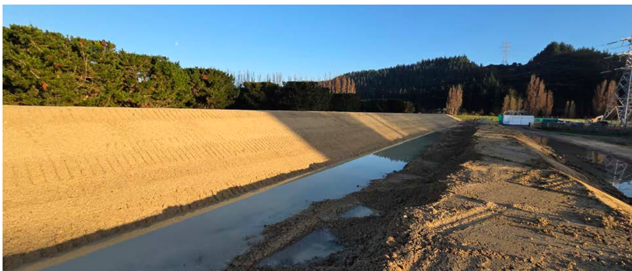
Pictured above: The industrial stopbank that will provide better flood protection for Pan Pac and our industrial neighbours Transpower and Contact Energy.
