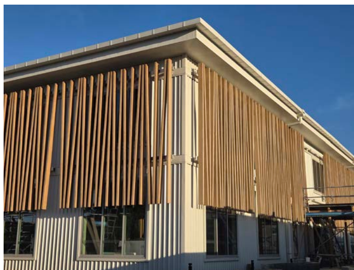
Pictured left: The exterior of the new office building of the Central Support Hub. The building has been clad in architecturally-designed shade fins produced by our customer Abodo timbers.
